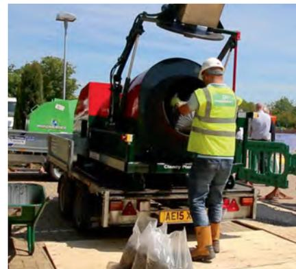
and utility clients across the country with a view to rolling out further machines towards the end of the year. The Roadmender allows first-time permanent, high quality repairs with polymer modified materials offering flexibility to gangs to carry multiple different mix designs on board to suit their needs.
