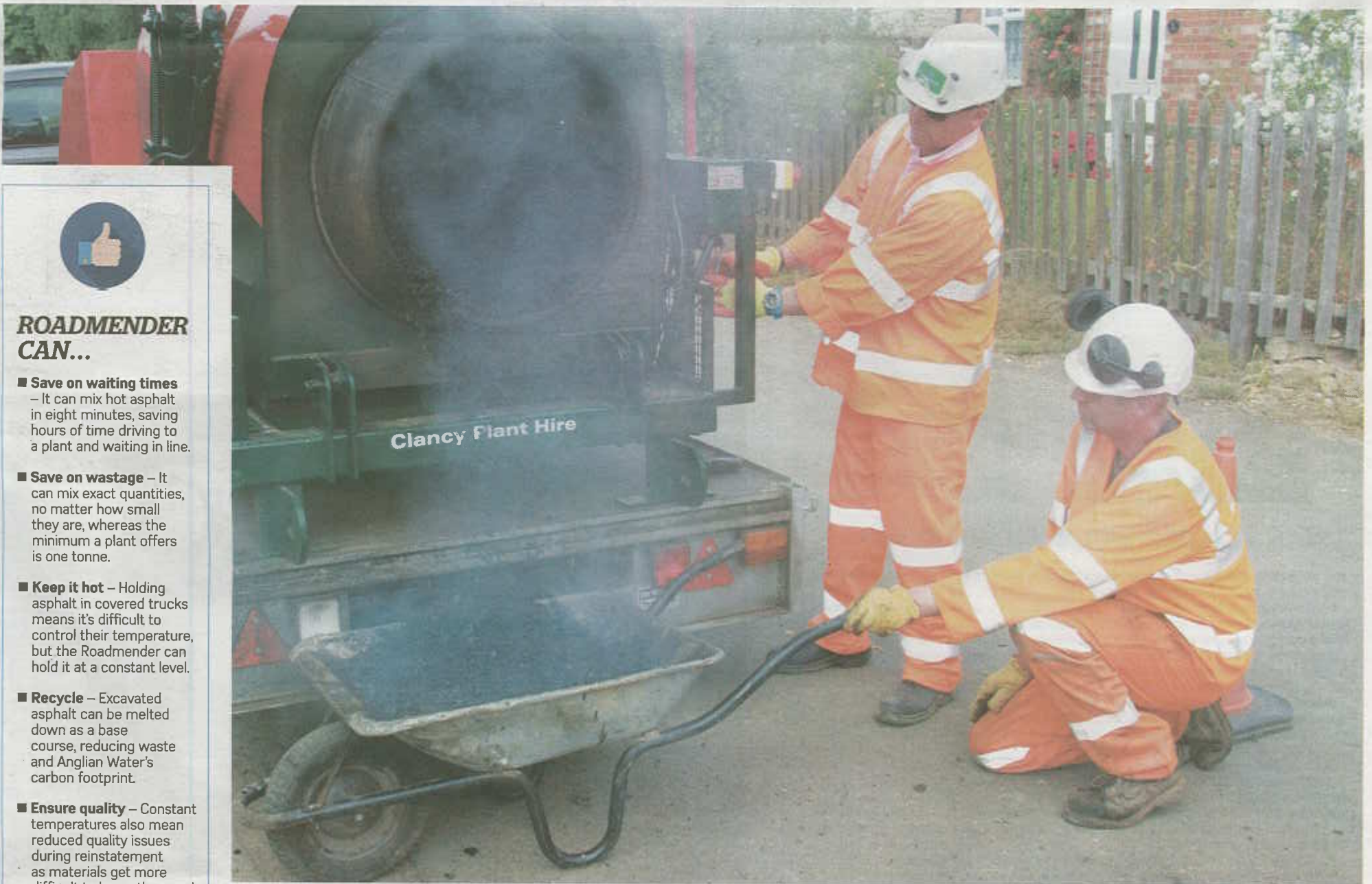
Hot and steamy: Technicians from Canwick Water Recycling Centre using the new Roadmender to repair a road in Rowston, near Lincoln
